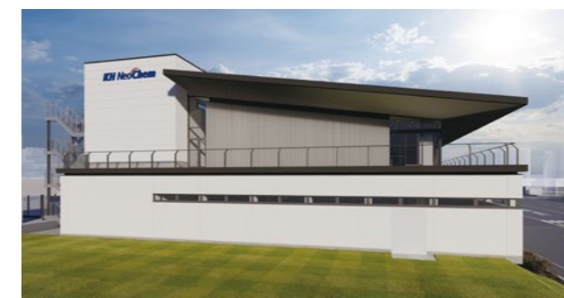
Building for quality control in Yokkaichi Plant, completion image
